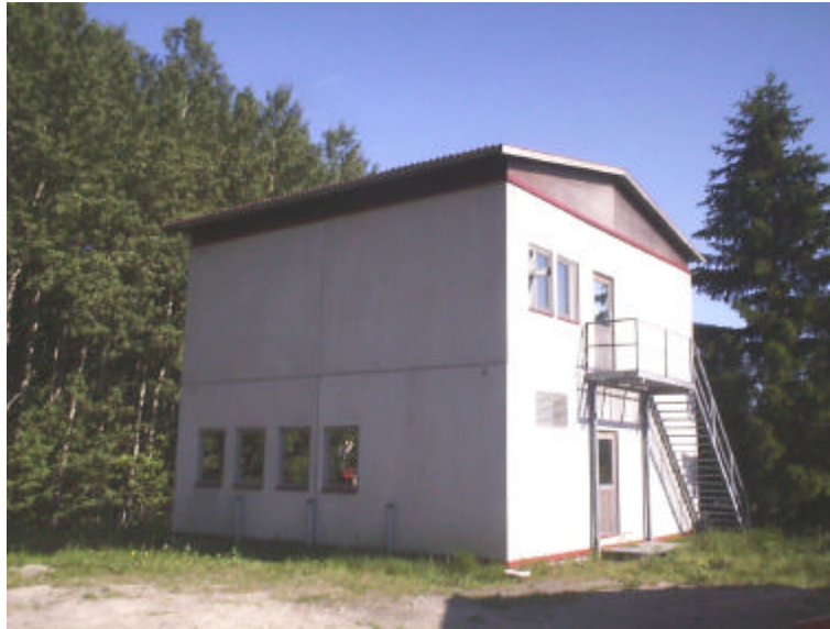
Figure 69: View of the experimental METOP-building (N and W facade)
