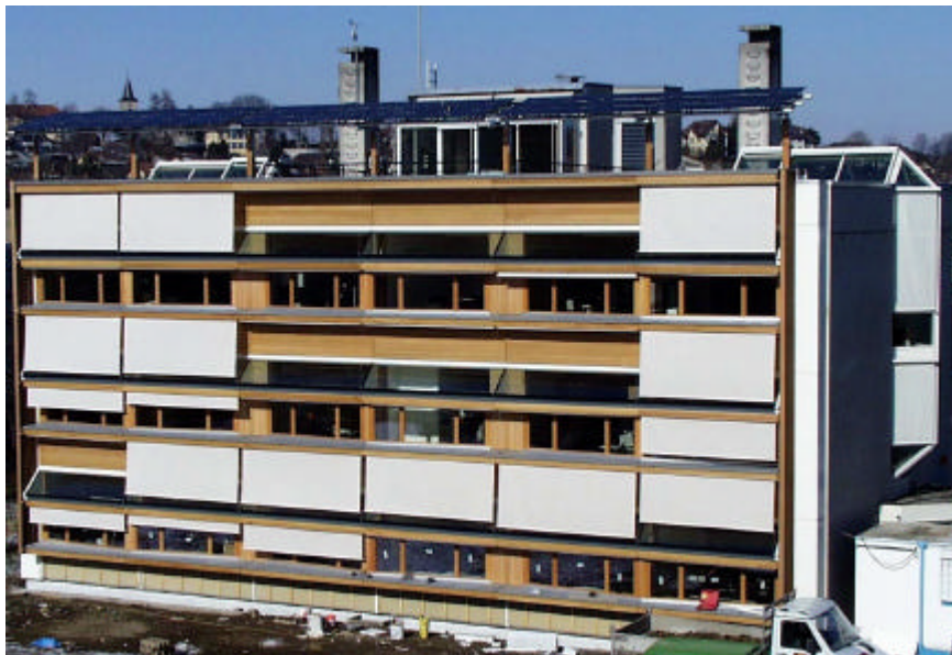
Figure 65: View of the south facade of LESO building
